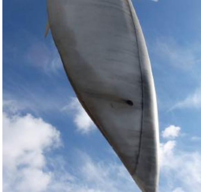
(b) Trailing Edge Blowout
