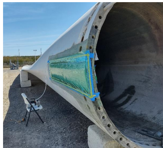
(c) Finished and Bagged First Sequence
