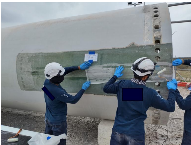
(b) Applying the First Layer of Laminate
