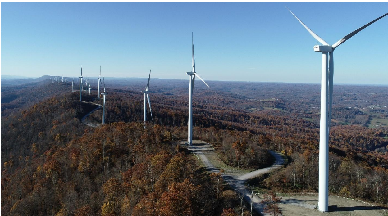
Figure 6: AES Laurael Mountain Wind Farm Facility, West Virginia
