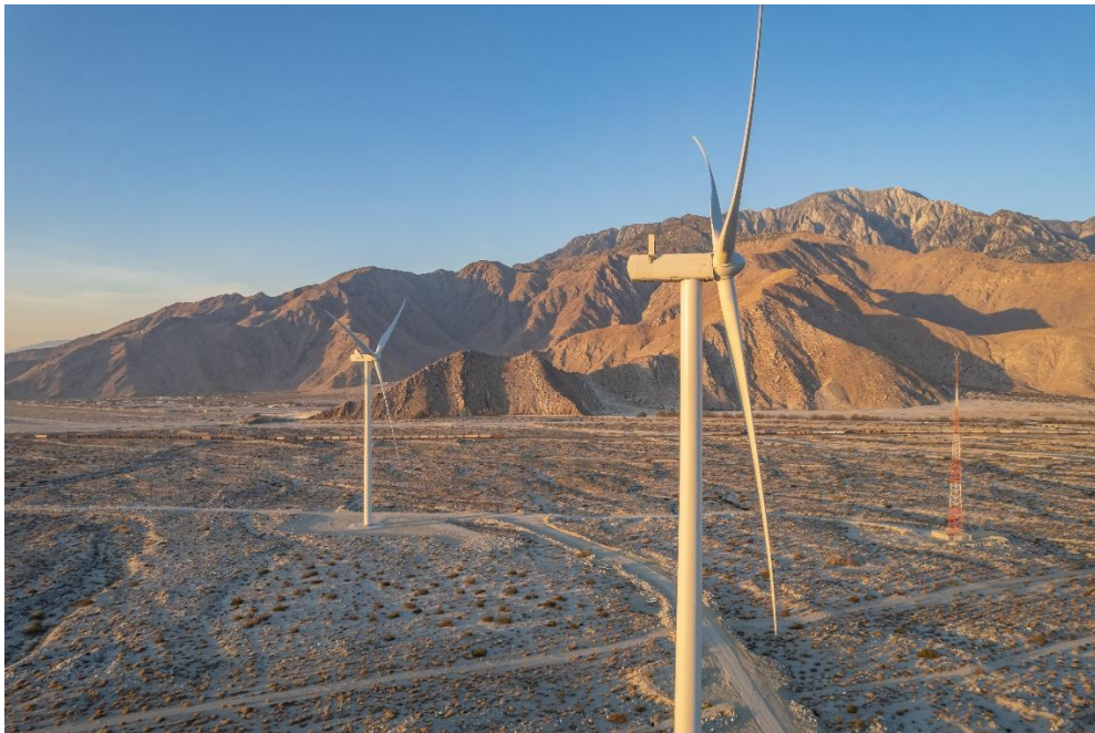
Figure 5: AES Mountain View Wind California
