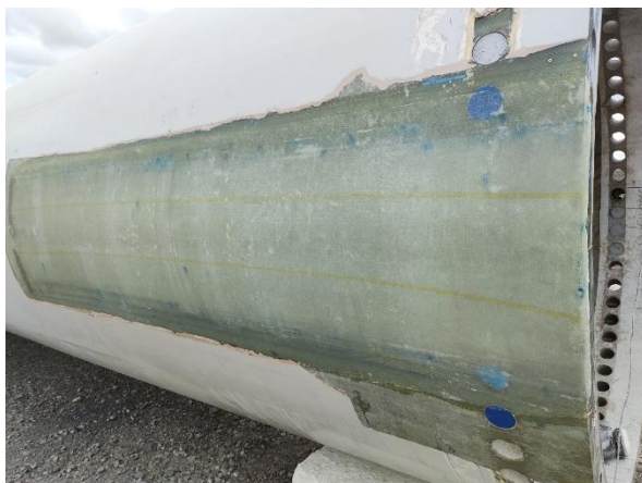
(a) Sanding of the Finished & Cured Laminate
