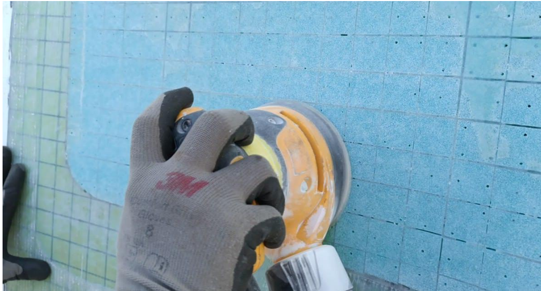
Figure 25: Example of the Final Sanding of a Glass Repair over Foam Core
