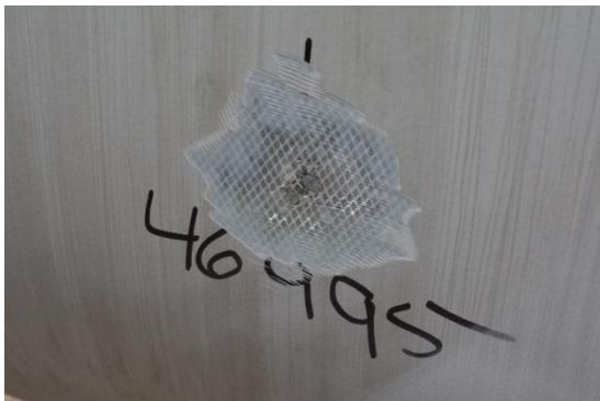
(a) Removal of Top Coat
