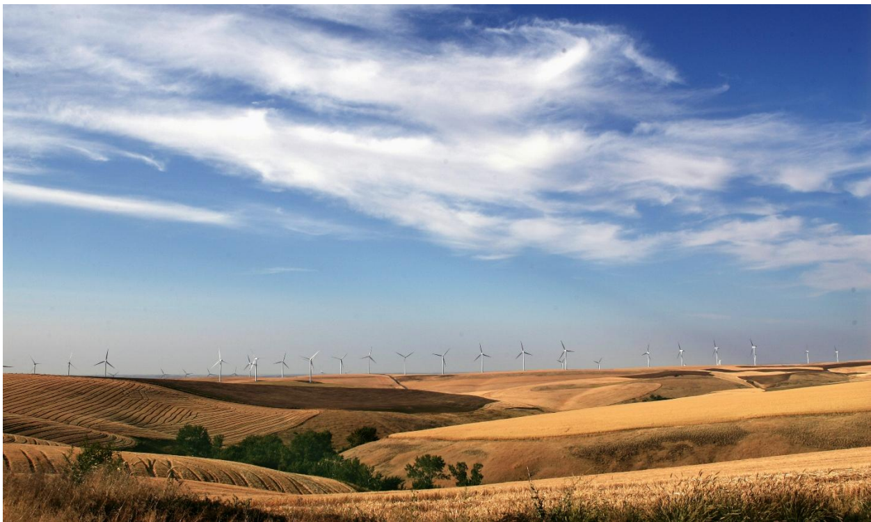
Figure 1: Hopkins Ridge Wind Farm
