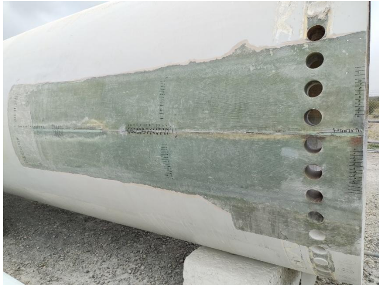
(a) Marking the Lamination Schedule
