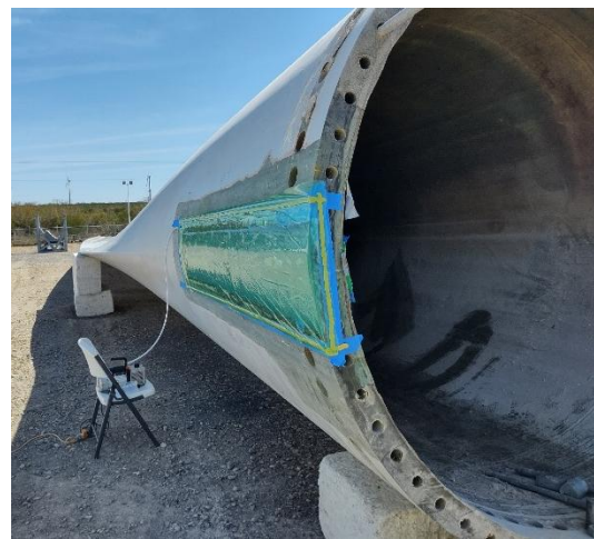
(c) Finished and Bagged First Sequence
