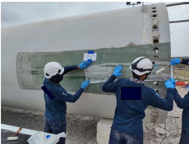
(b) Applying the First Layer of Laminate
