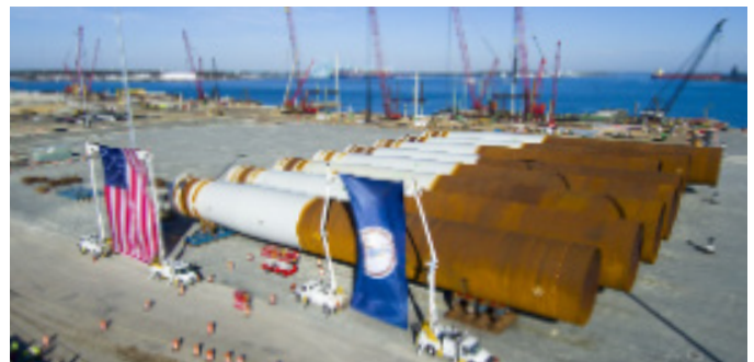
Port of Virginia helps prepare components ahead of installation at the Coastal Virginia Offshore Wind Project.
