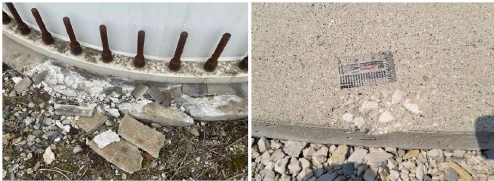
Figure 11. Structurally significant pedestal spalling in left photo and minor debris/impact pedestal spalling in right photo.
