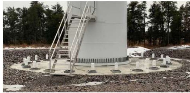
Figure 4. Rock anchor foundation in service in left photo, and three-dimensional image illustrating the design elements of the rock anchor foundation in the right photo.
