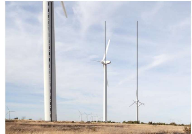
Figure 21. Example of a foundation out of level resulting in visually observable tower tilt compared to neighboring turbines. Solid vertical lines are drawn representing two plumb and vertical towers to the right whereas the tower on the left has a tower centerline, shown with a dashed line, that is not plumb.
