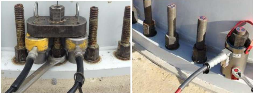
Figure 19. Jack and plate tension method setup shown in left photo and bolt tensioner on an anchor bolt in the right photo [ITH Bolting Technology, www.ith.com ].
