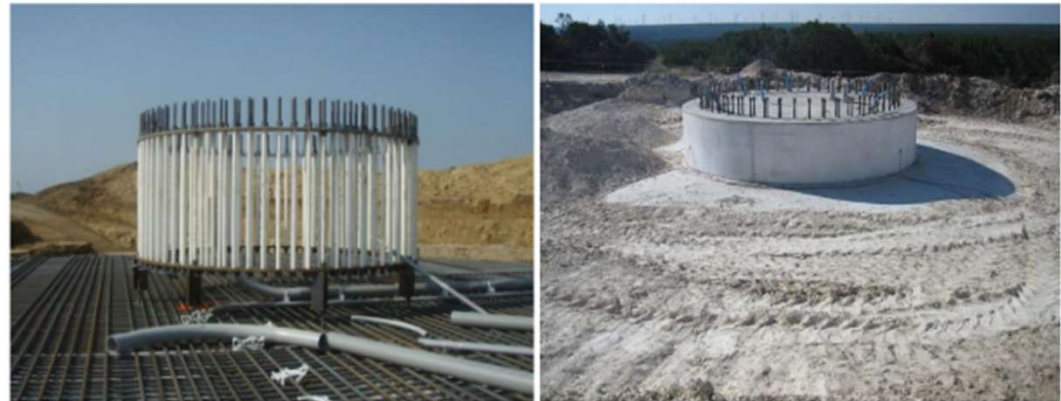
Figure 7. Anchor bolt/embedment plate assembly prior to concrete placement shown in left photo and fully constructed foundation in the right photo.
