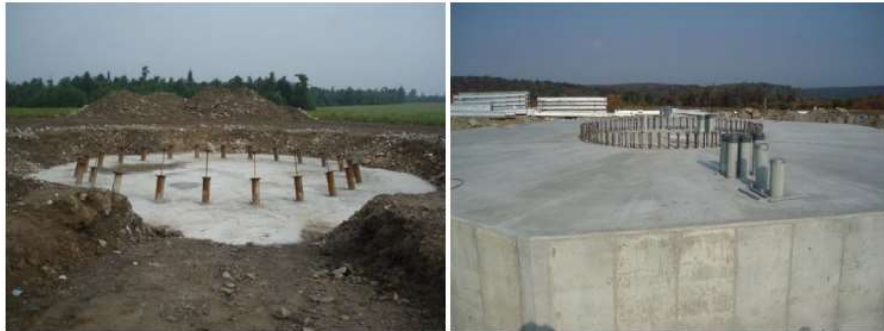
Figure 5. Pile supported cap foundation in construction in left photo and completed foundation in right photo.
