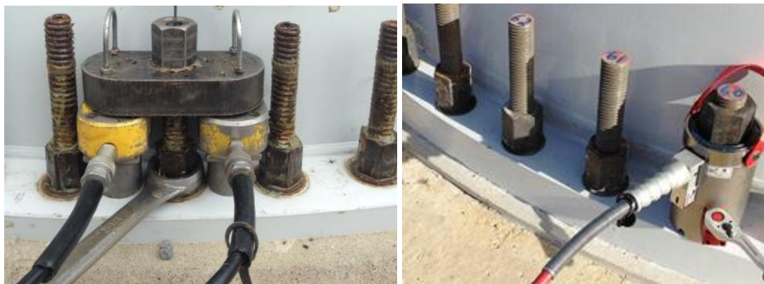
Figure 19. Jack and plate tension method setup shown in left photo and bolt tensioner on an anchor bolt in the right photo [ITH Bolting Technology, www.ith.com ].
