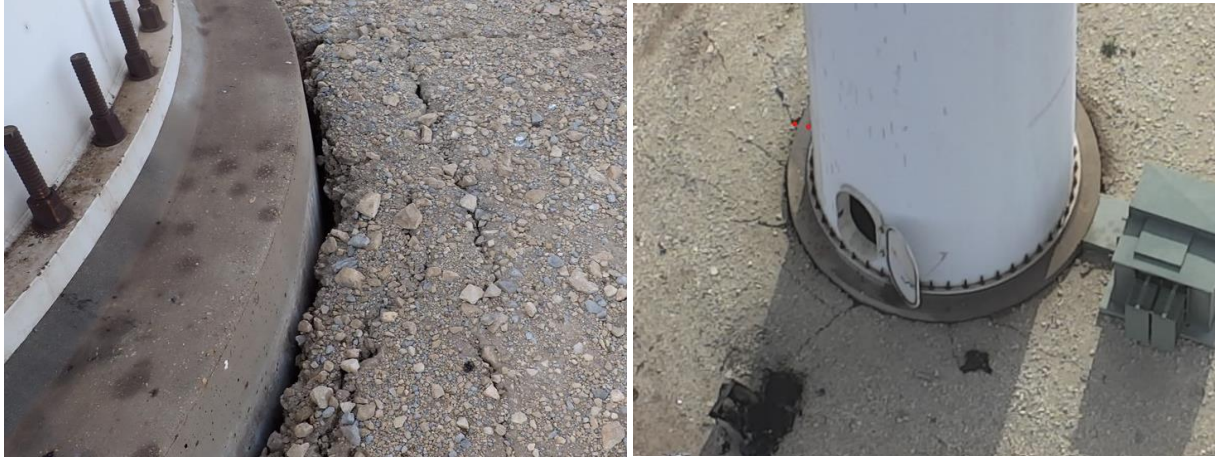
Figure 18. Gap between pedestal and backfill from close-up in left photo and aerial view of foundation soil cracking in right photo.
