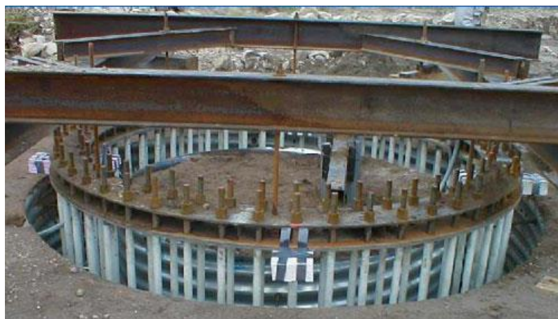
Figure 3. Tensionless tube foundation anchor cage ready for pour in left photo, and three-dimensional image illustrating the design elements of the tensionless tube foundation in the right photo.
