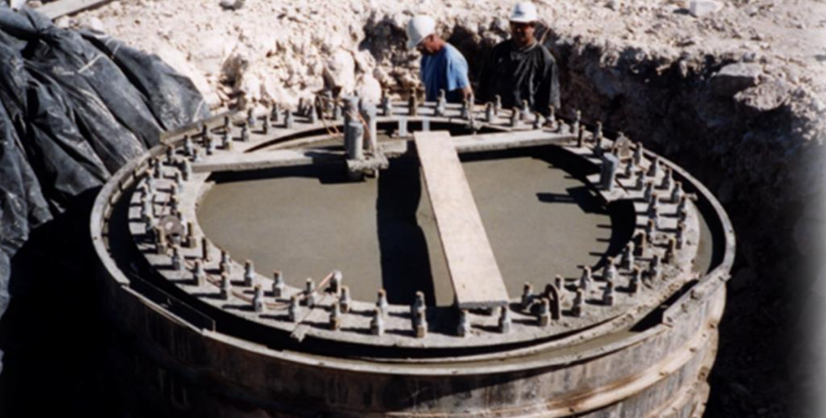
Figure 6. Rock socket foundation in construction prior to backfill.
