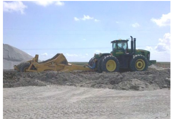
Figure 4.1: Removing Top Soil
