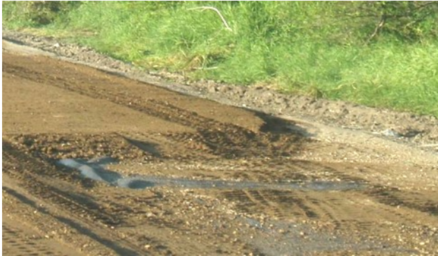
Figure 4.2: Installing Geotextile Fabric
