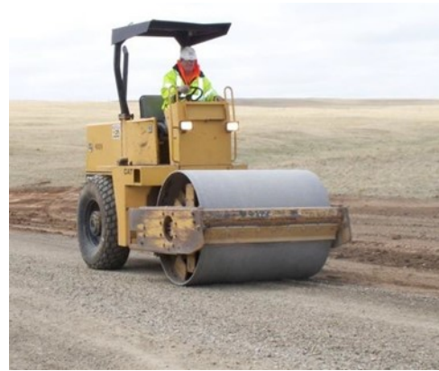
Figure 4.4: Compacting Road Base
