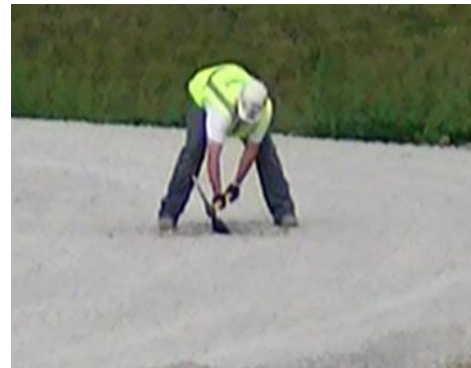
Figure 4.5: Performing QC Check on Gravel Installation
