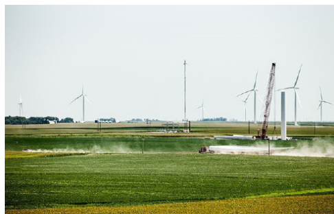
Highland Wind Farm construction, O'Brien County, Iowa
