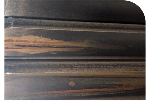
Figure 5: False Brinell Mark with Fretting Corrosion
