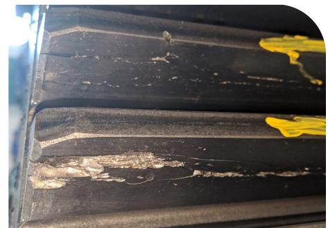
Figure 12: Example of two cracked teeth, one has progressed enough to remove areas of the surface material, the other is not as progressed.
