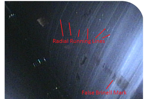
Figure 17: Bearing roller with typical radial running lines and a false Brinell mark. Debris dents can also be seen on the roller.
